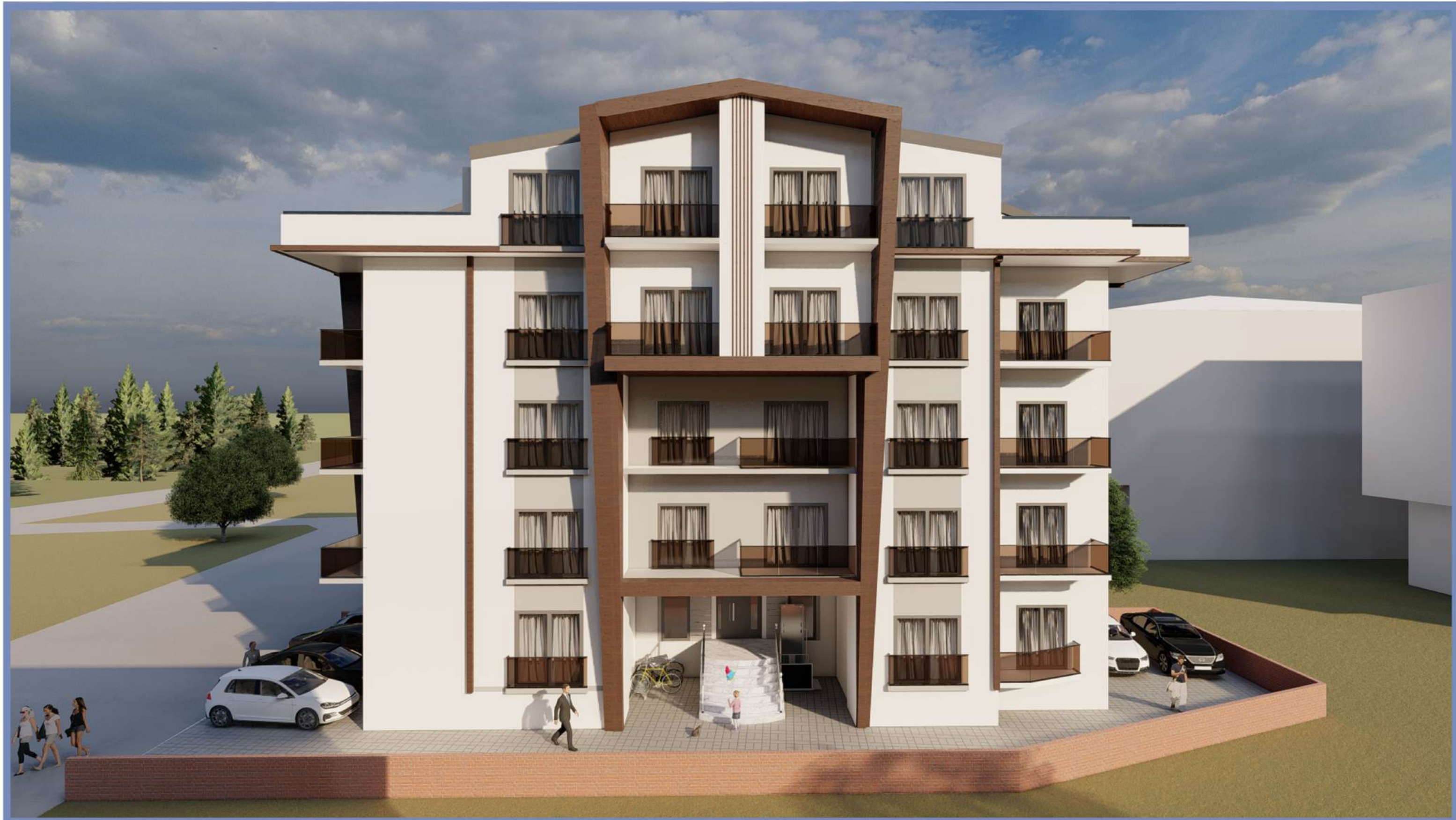
BENGI APARTMANI B BLOK
